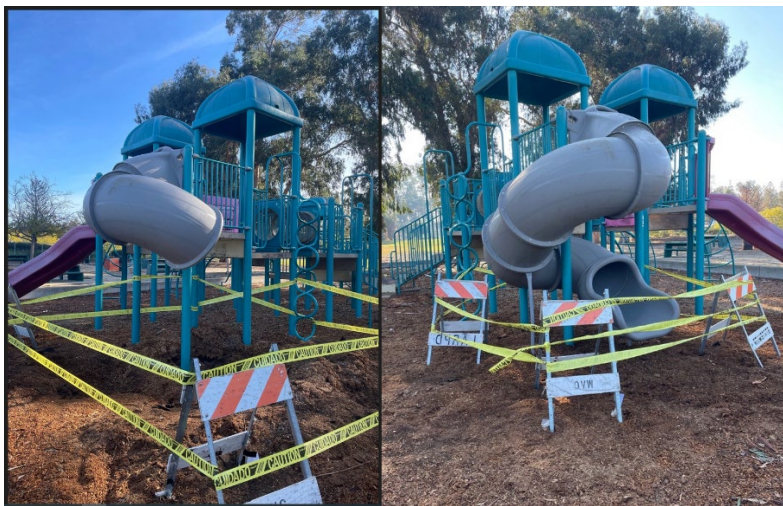
Hagemann Slide Installation Before Hagemann Slide Installation After
