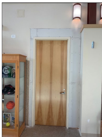
RLCC Door Installation
