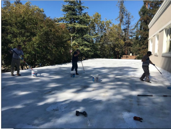
R.E. Merritt Building Roof Repair
