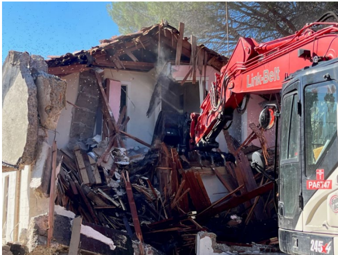
Ledford House Demolition
