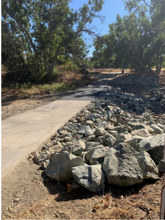
Completed Trail Repairs
