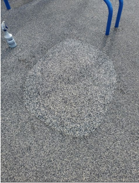
Altamont Creek PIP After Repair
