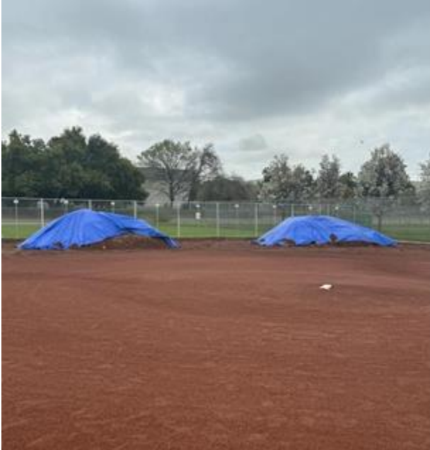
Bill Payne infield renovation project.
