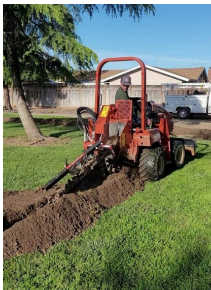
May Nissen Dog Park Irrigation installation
