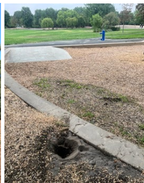
Tex Spruiell Lateral & Irrigation Mainline Repairs
